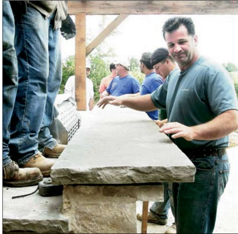
DIY Network's "Inside Out" co-host Dean Marsico (right) looks over a 12-foot, 2-inch-thick blue stone countertop weighing 600 pounds during a patio remodel in Drumright. SHERRY BROWN/Tulsa World
